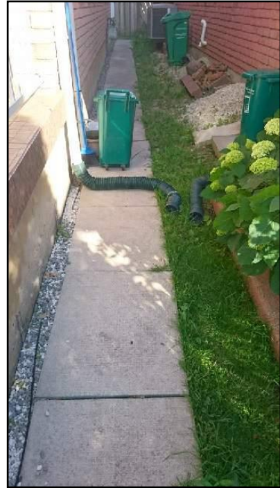
6. Away from building
