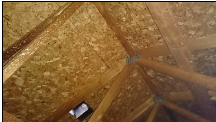
14. Roof and soffit vents
